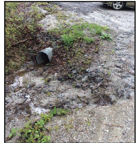
Sediment and gravel from this driveway above is washing directly into the municipal ditch system and can travel directly into Lake Champlain
