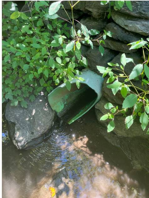
Figure 1. Outfall 11 located on Barlow Street, discharging to Stevens Brook.
