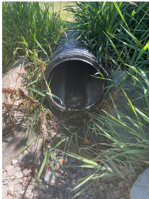
Figure 8. Outfall 54 in the back of the St. Albans City Elementary School.
