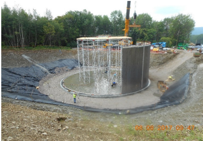
Example Concrete Water Storage tank during construction.
