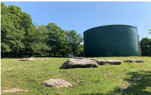
Aldis Hill Water Storage Tank Site & Existing 1.0 Million Gallon Water Storage Tank
