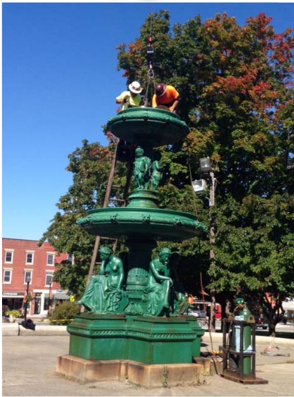
Workers from Robinson Iron dismantle the fountain
